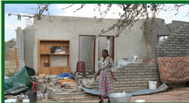
HOMELESS: One of the several houses in Dumphries C was left roofless after the storm.
