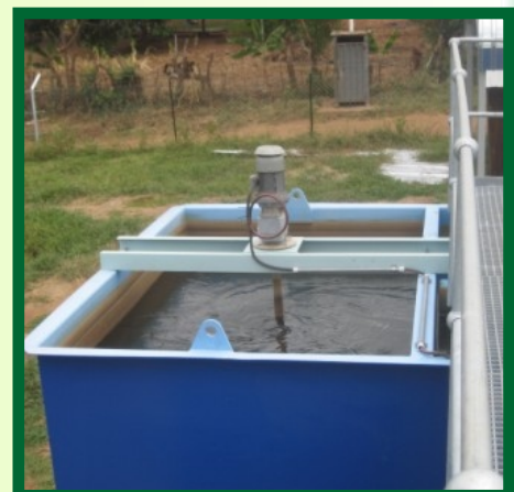
MIG INFRASTRUCTURE: Construction of the Water Treatment Plant at Langeloop in the Nkomazi Municipality
