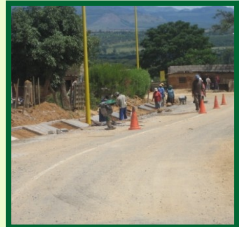
REHABILITATION: An MIG road construction project in Barberton
