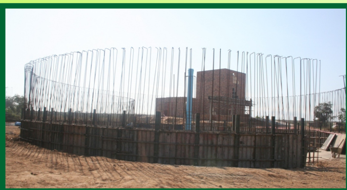
WATER: Construction of a water plant at Block C
